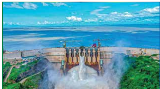
Julius Nyerere Hydro Electric Power Project after switching on all nine turbines
