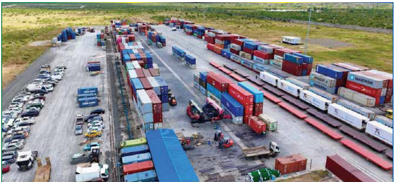
Container operations at Kwala Dry Port – boosting cargo efficiency and reducing port congestion
